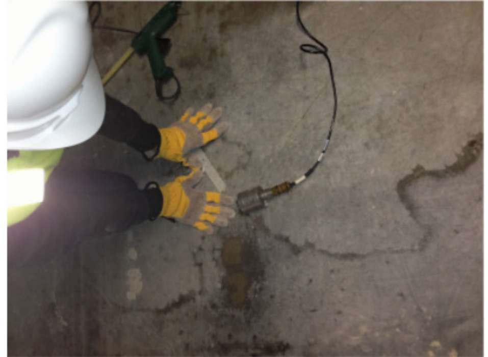
Adhering grid-point location plates for accelerometers on test floor
