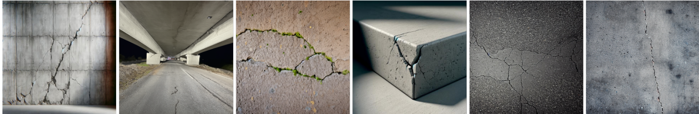
Figure 2: Synthesized crack images generated using the CRKGEN.
