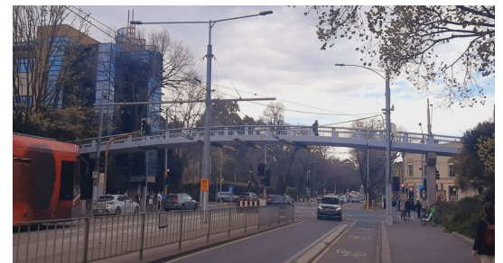
Figure 1 Pedestrian bridge over Swanston Street, Parkville, Australia
